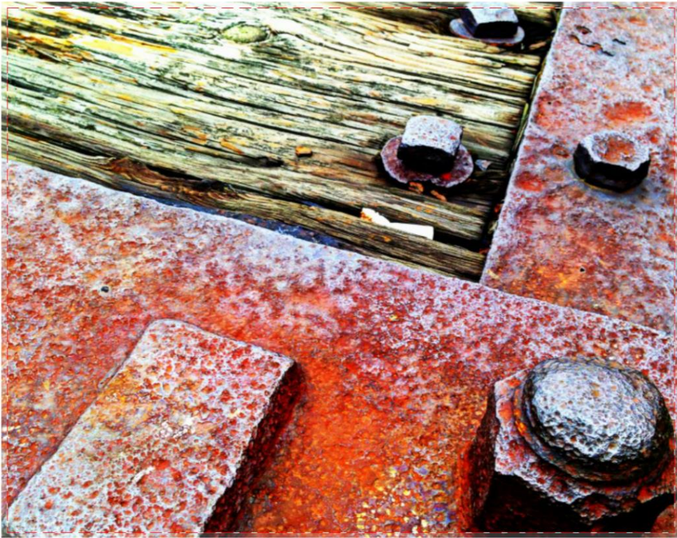
Rusted Beam Golden 11 x 14 Wall Panel $100
